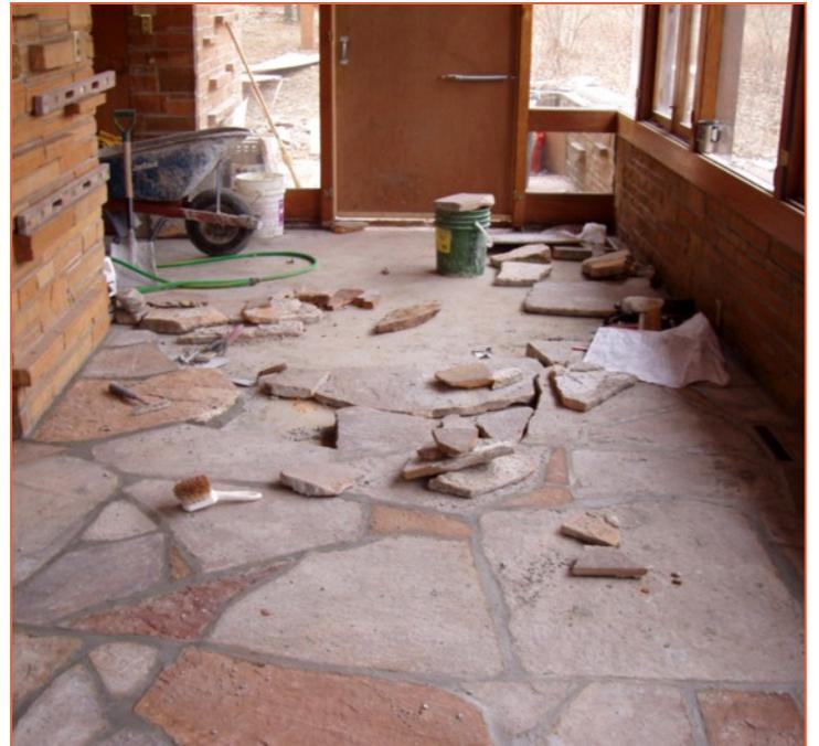
*Reinstalling flagstone flooring after heating tube replacement 2006*
