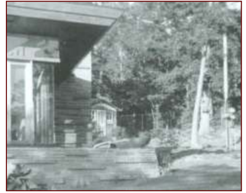
Original Garden Shed and Power Pole
